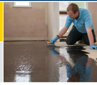
**SETCRETE™ RAPID SET DPM** is a solvent free, two part epoxy resin system which cures to provide a damp proof membrane. SETCRETE™ RAPID SET DPM provides a barrier to residual construction moisture and rising damp, preventing moisture from adversely affecting subsequent floorcovering installations. The product is applied in one coat and has a curing time from just 3 hours, allowing early installation of floorcoverings in fast-track building programmes.
